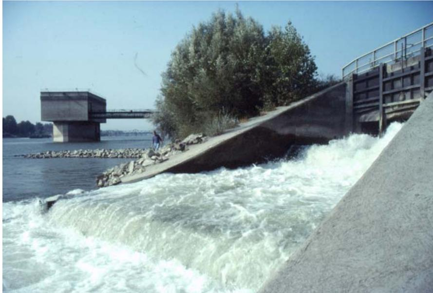
Fig.1: surface discharge of the Donaustadt cooling water ( $8.6 \text{ m}^3/\text{s}$ ) prior to the construction of the River Danube hydro power plant Vienna-Freudenau
