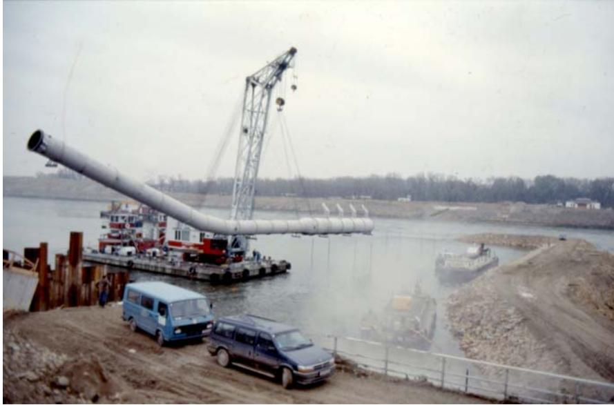
Fig.3: diffuser piece moved by ship crane
